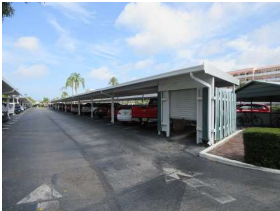
Photo No. 23 – View of small storage area under carports for trash cans and bike racks.
