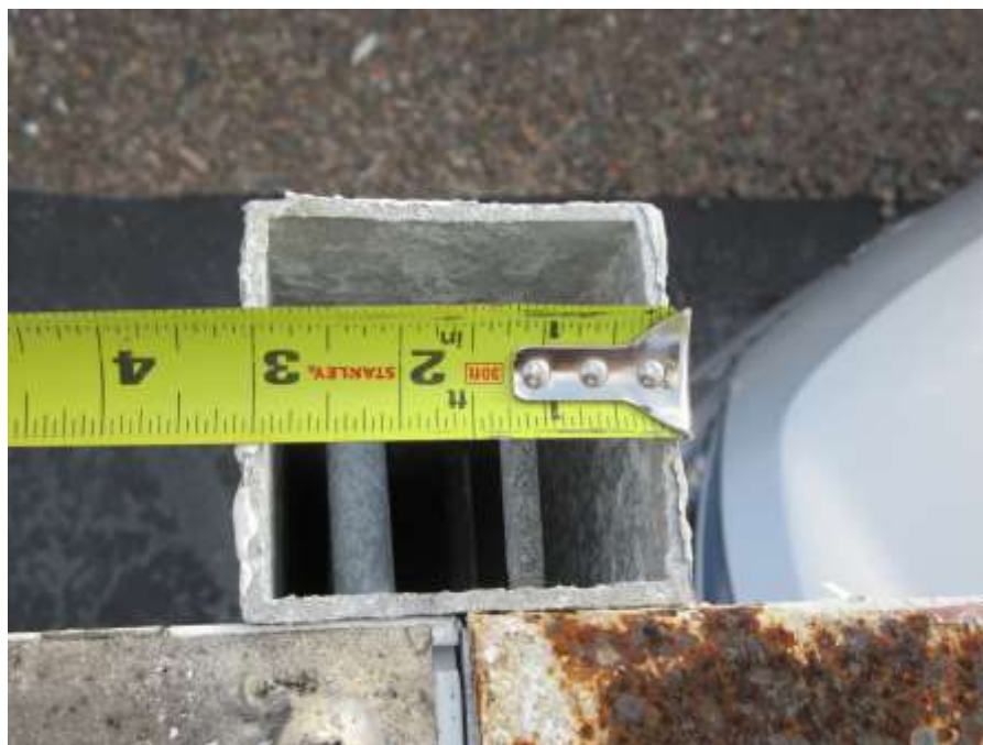
Photo No. 9 – 3” square tube columns built in the concrete foundation pads
