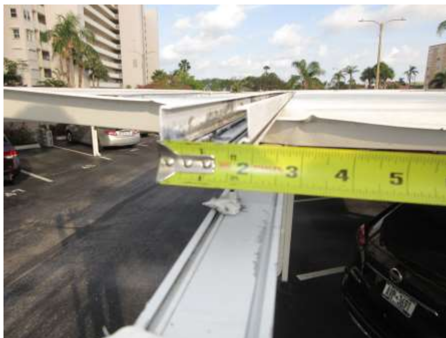
Photo No. 10 – Typical 2”x1” Screen Channels
