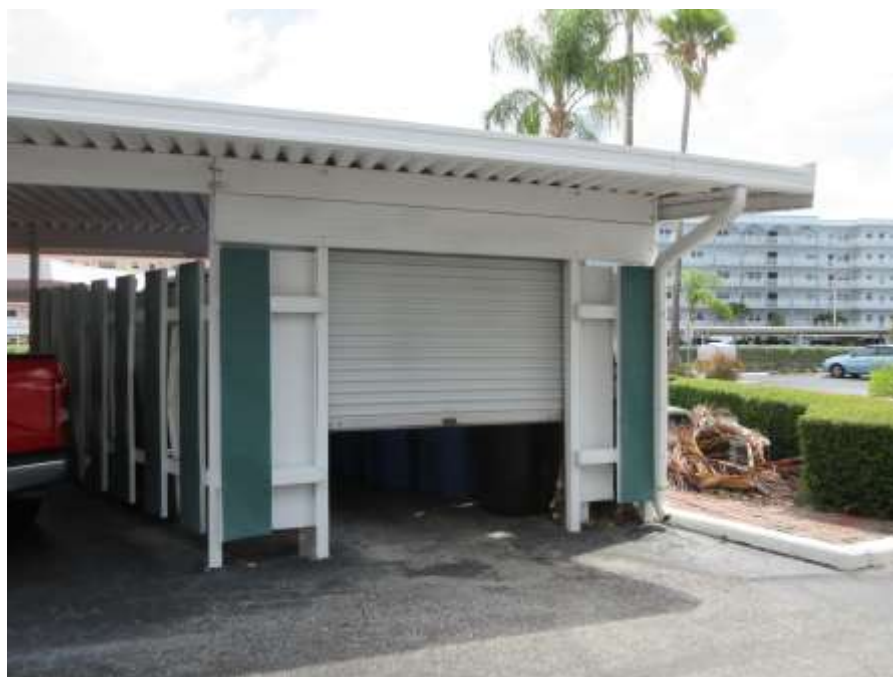
Photo No. 26 – Storage area in bay #2 for trash cans.
