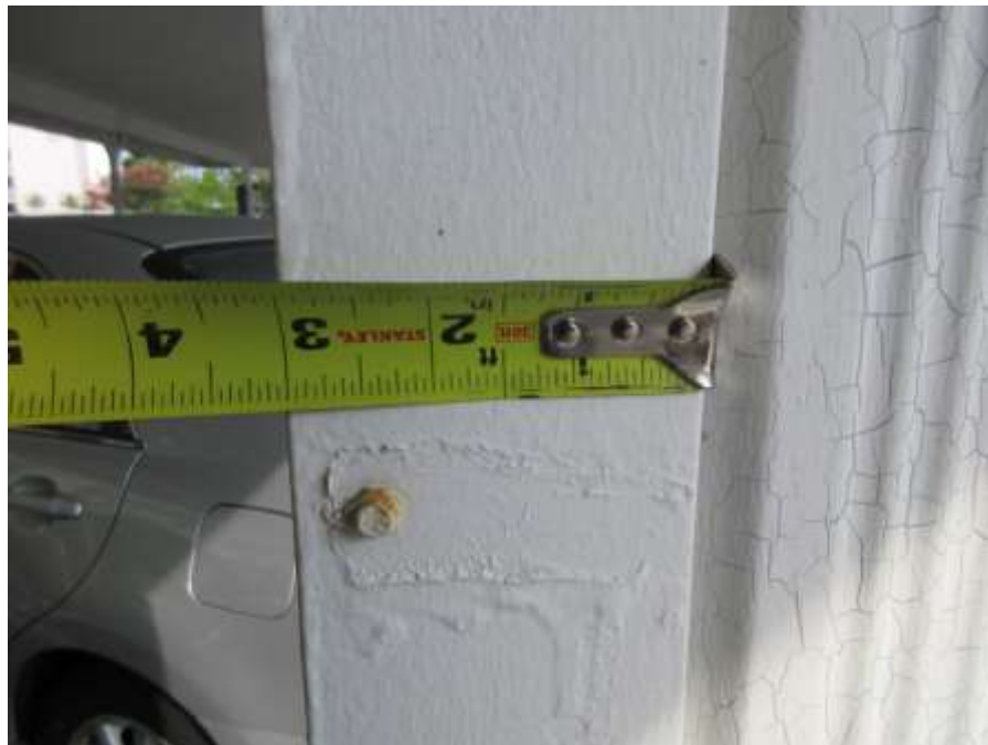
Photo No. 14 – 3-in steel tubes used for column members.
