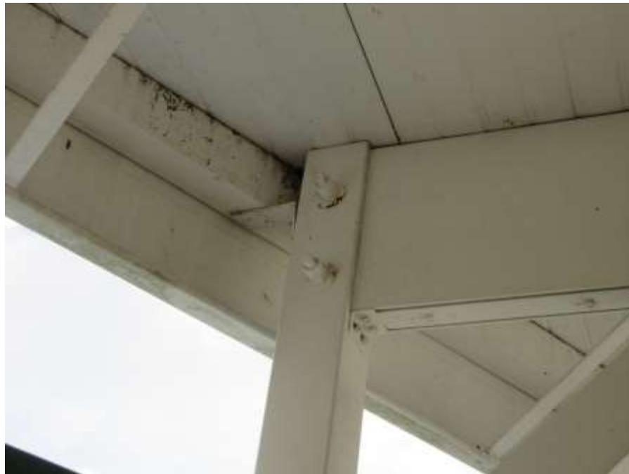
Photo No. 12 – Steel framing connection with bolts.
