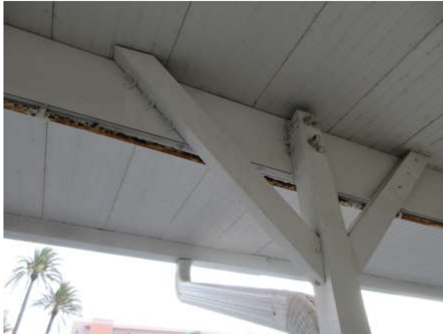
Photo No. 13 – Simple Steel framing connection with diagonal bracing.
