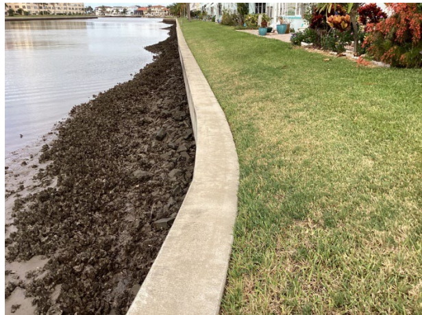
Concrete bulkhead
