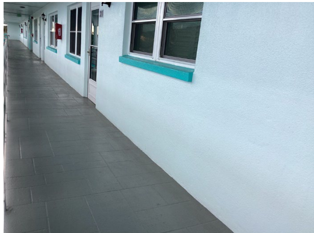
Stucco wall finishes at the breezeways
