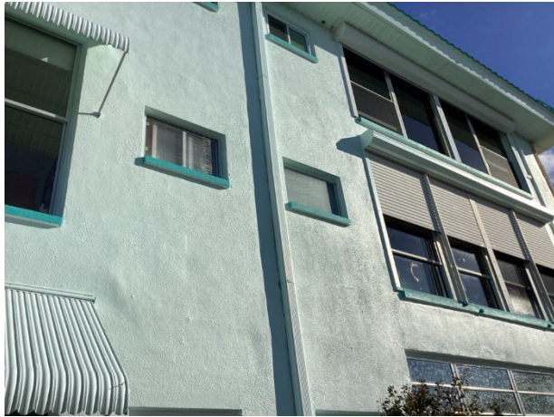
Stucco wall finishes
