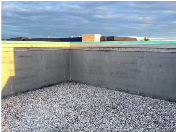
Parapet walls overview
