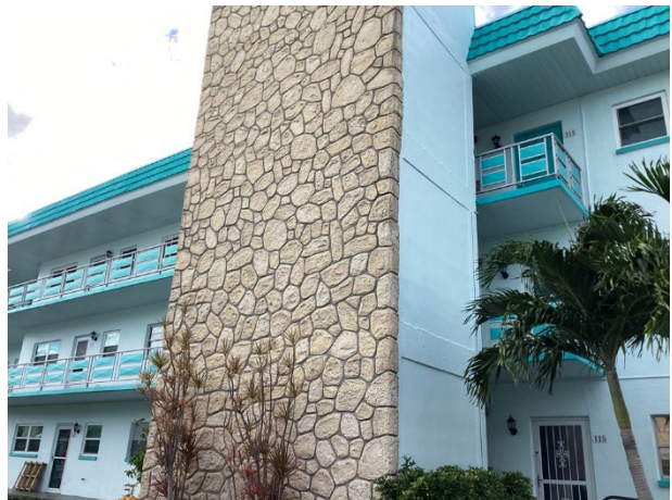
Masonry wall overview
