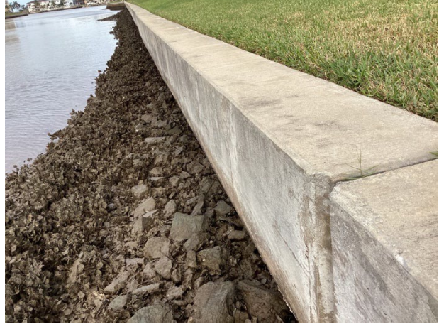
Concrete bulkhead
