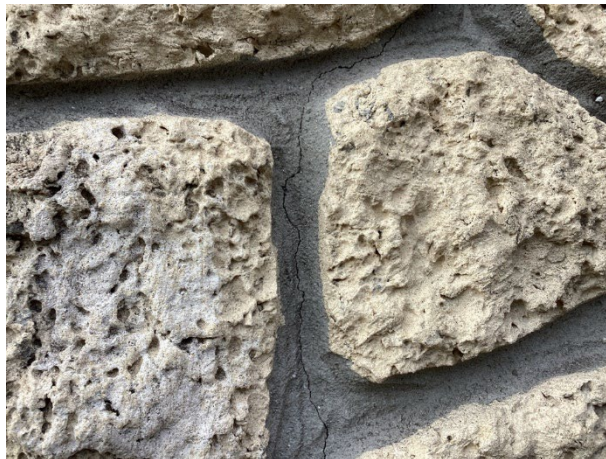
Mortar cracks
