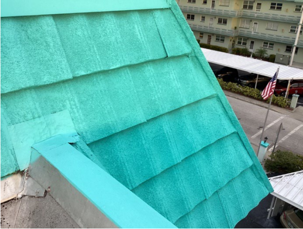
Metal mansard roof
