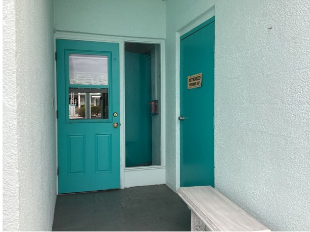
Common area doors
