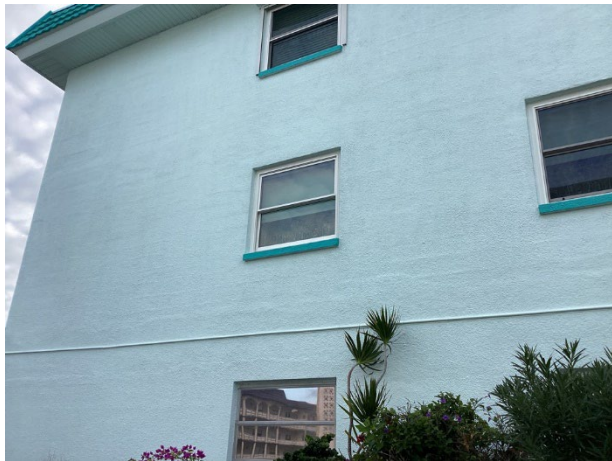
Stucco wall finishes
