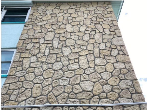
Masonry wall overview
