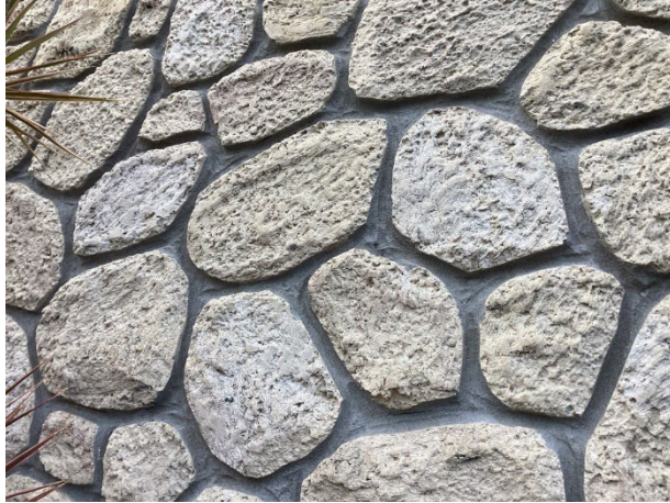
Masonry wall overview
