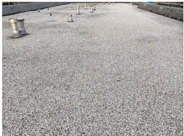
Built-up roof overview
