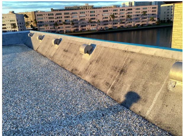
Parapet walls overview
