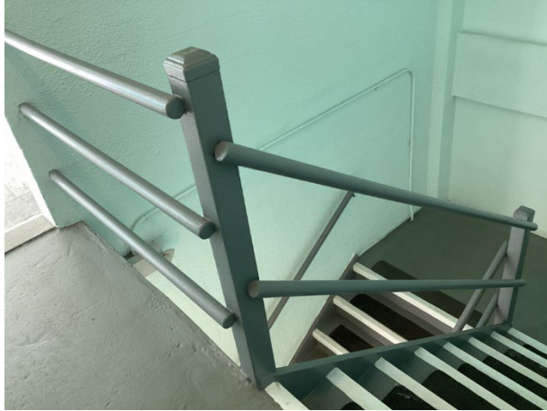
Staircase railings overview
