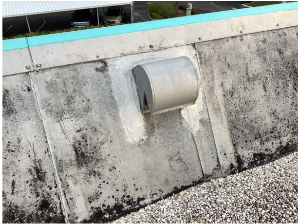
Patch repairs at the parapet walls
