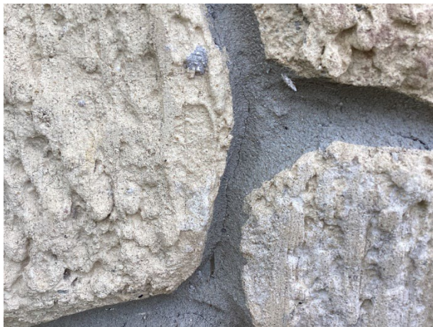
Mortar cracks
