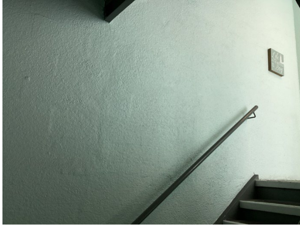
Stucco wall finishes at the stairwells
