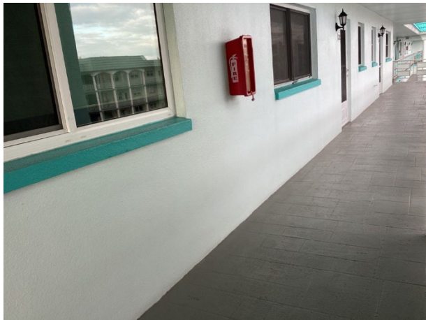
Stucco wall finishes at the breezeways
