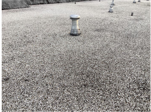
Built-up roof overview
