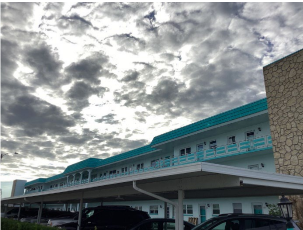
Metal mansard roof
