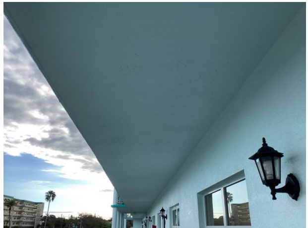
Breezeway underside overview
