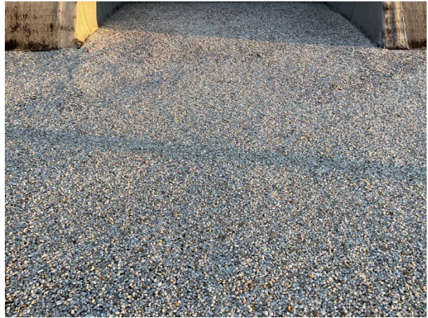
Built-up roof overview
