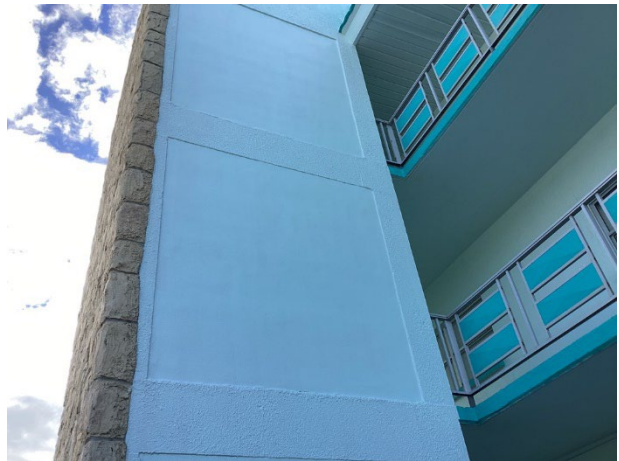
Stucco wall finishes
