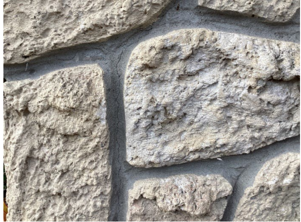
Mortar cracks
