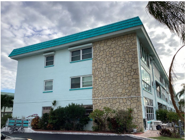
Side elevation of building
