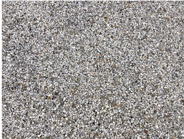
Built-up roof overview
