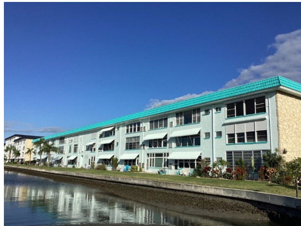
Rear elevation of building
