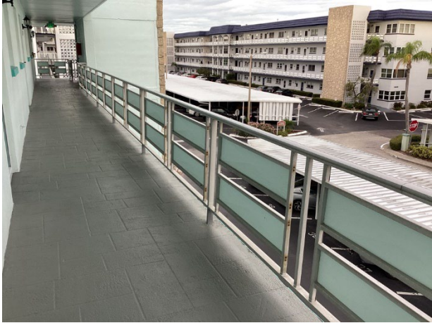
Metal breezeway railings
