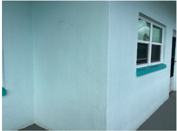
Stucco wall finishes at the breezeways
