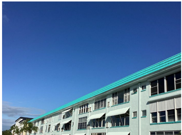
Metal mansard roof
