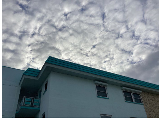
Metal mansard roof
