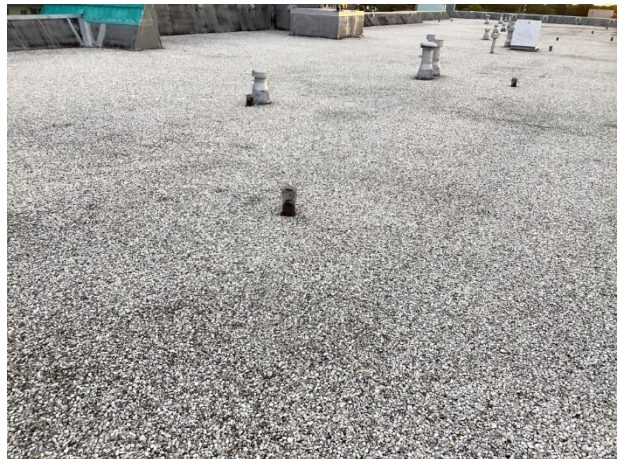
Built-up roof overview
