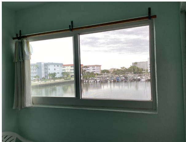
Window at the laundry room
