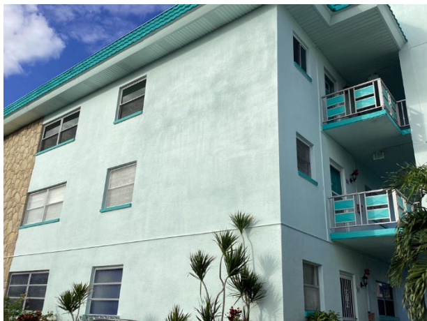
Stucco wall finishes
