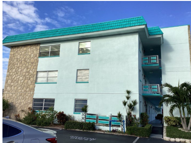
Side elevation of building
