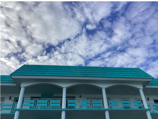
Metal mansard roof
