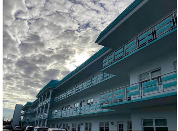
Metal breezeway railings
