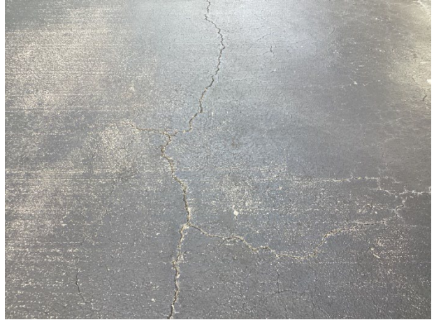
Pavement cracks
