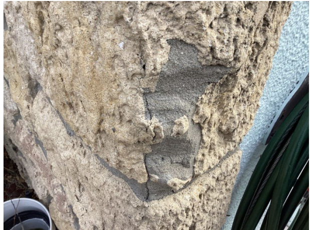
Mortar cracks
